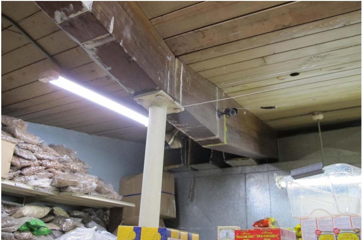
Fig. 84 – Interior, fourth and fifth bays (grocery store), detail of metal column and glue-laminated beam
