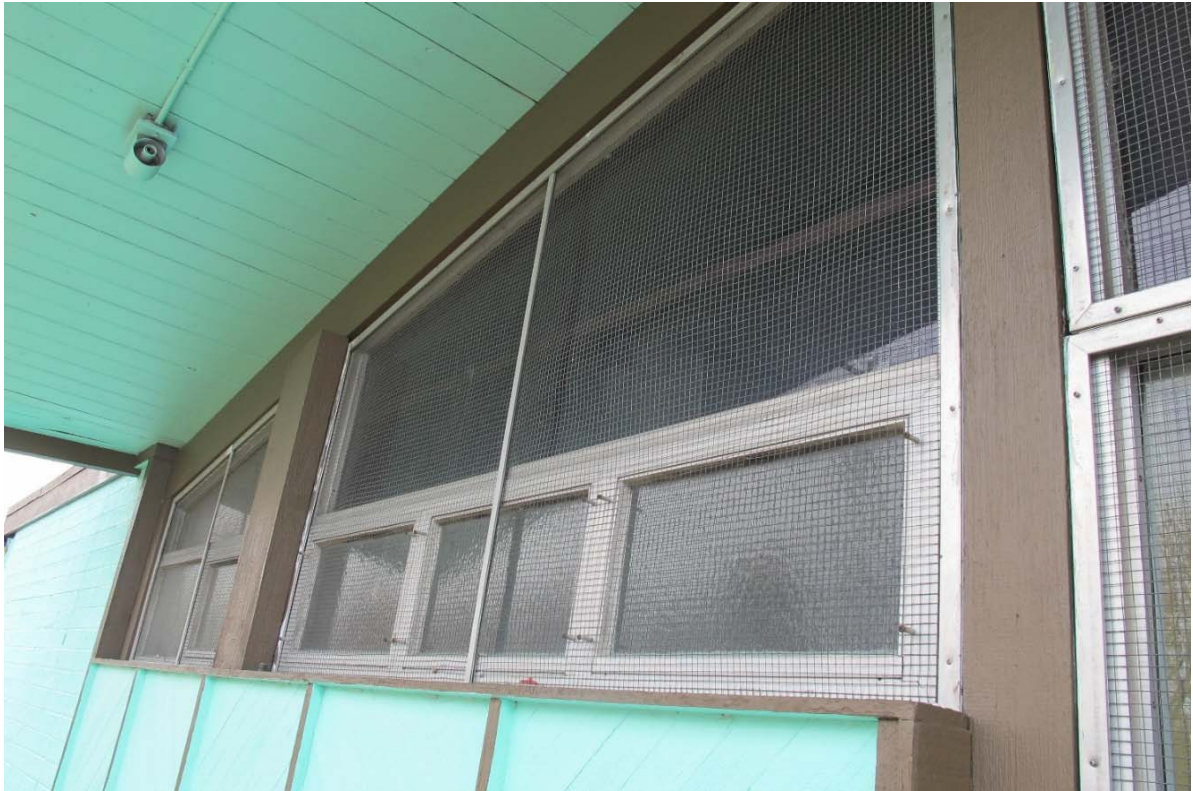
Fig. 53 – West elevation—first bay, detail of upper window
