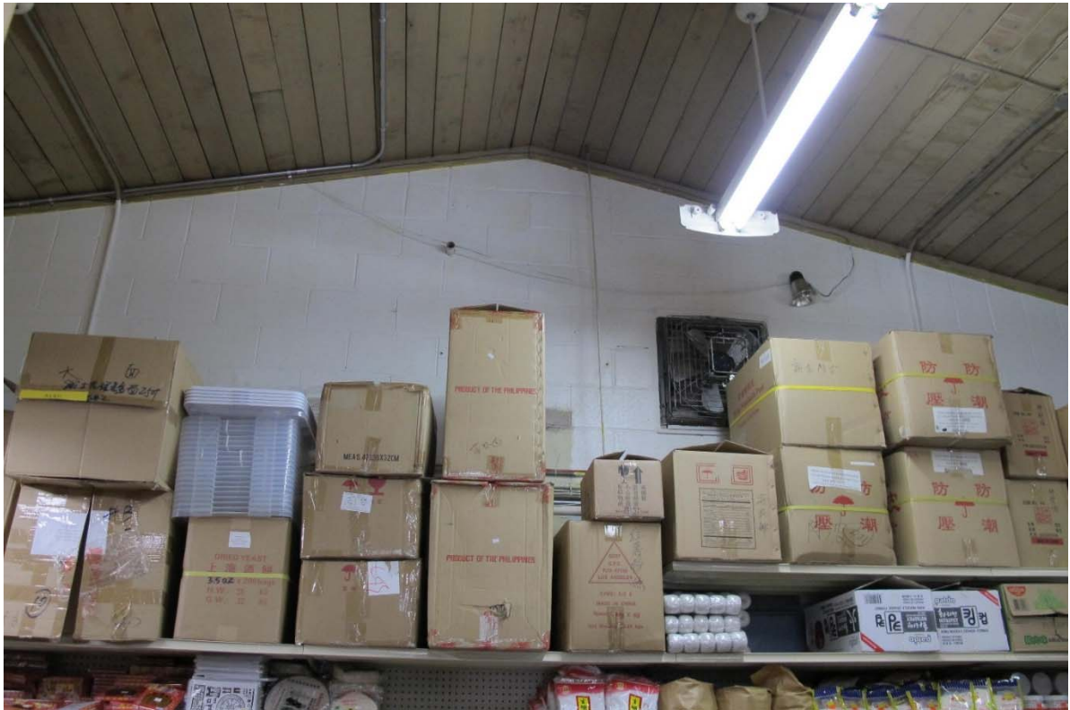
Fig. 76 – Interior, fifth bay (grocery store)
