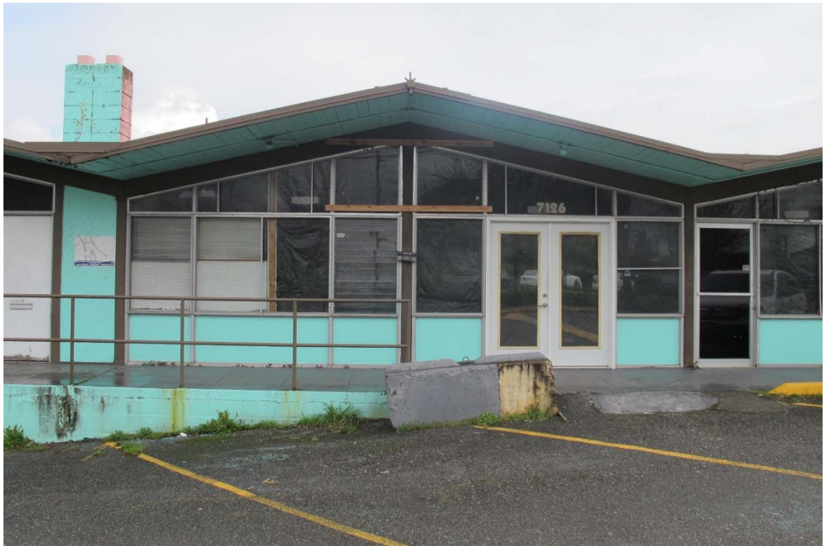
Fig. 57 – West elevation—second bay
