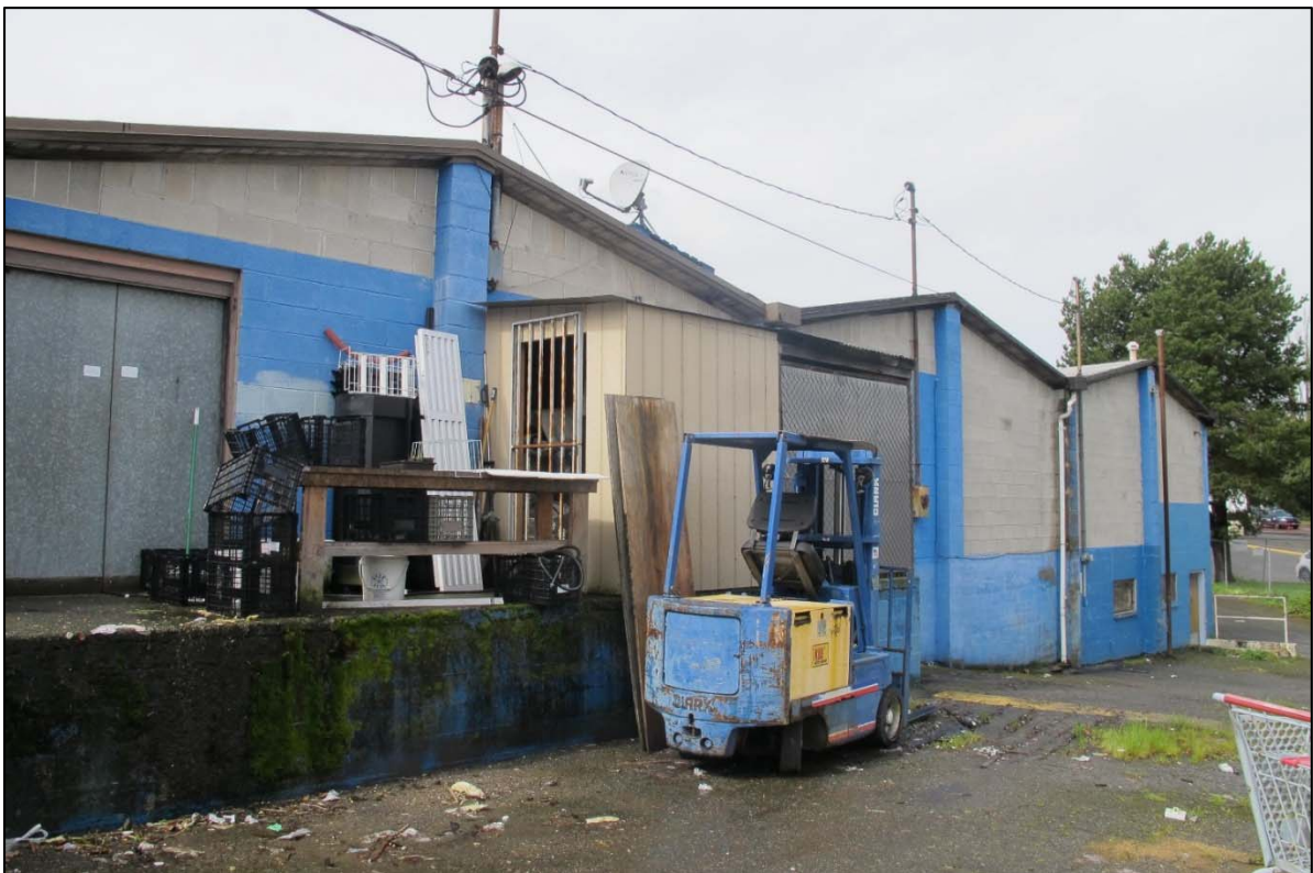
Fig. 42 – East elevation—fourth, third, and second bays
