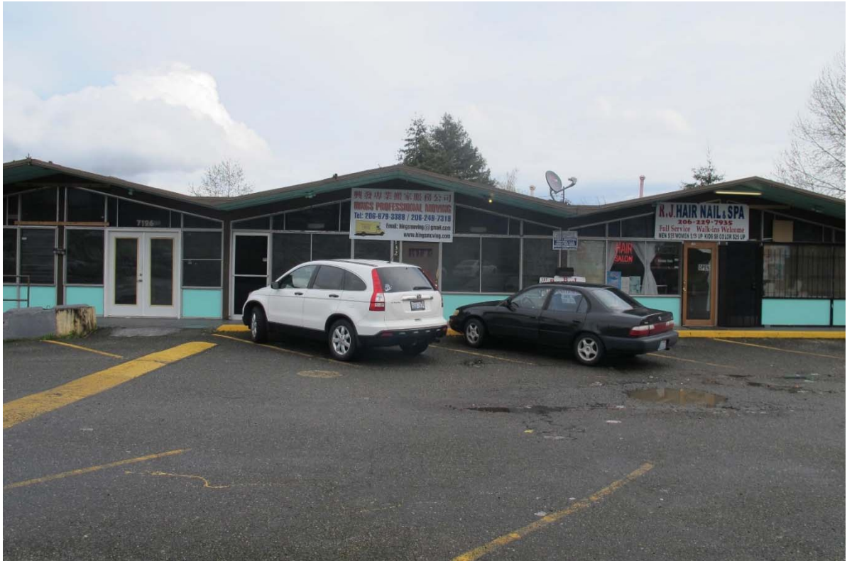
Fig. 63 – West elevation—second bay
