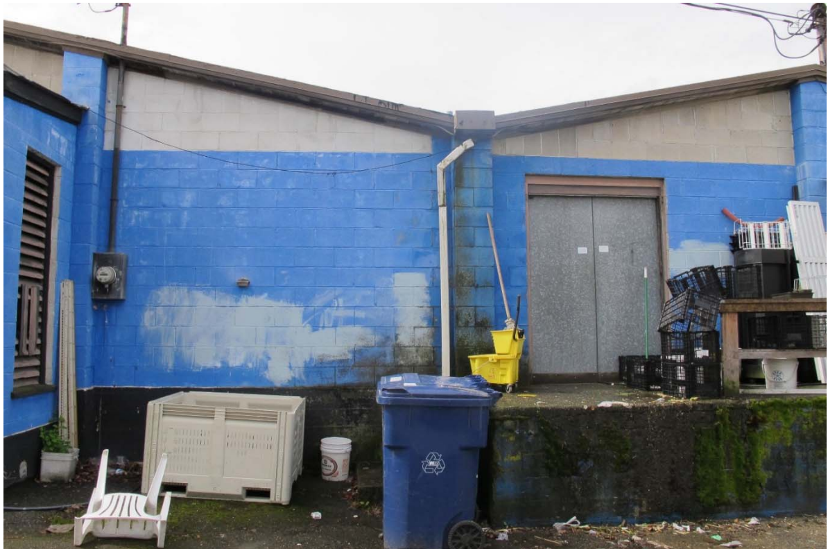
Fig. 41 – East elevation, south portion, view between fourth and fifth bays
