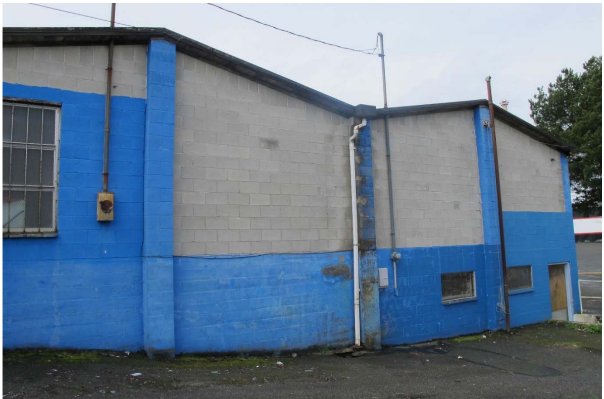
Fig. 44 – East elevation—third and second bays
