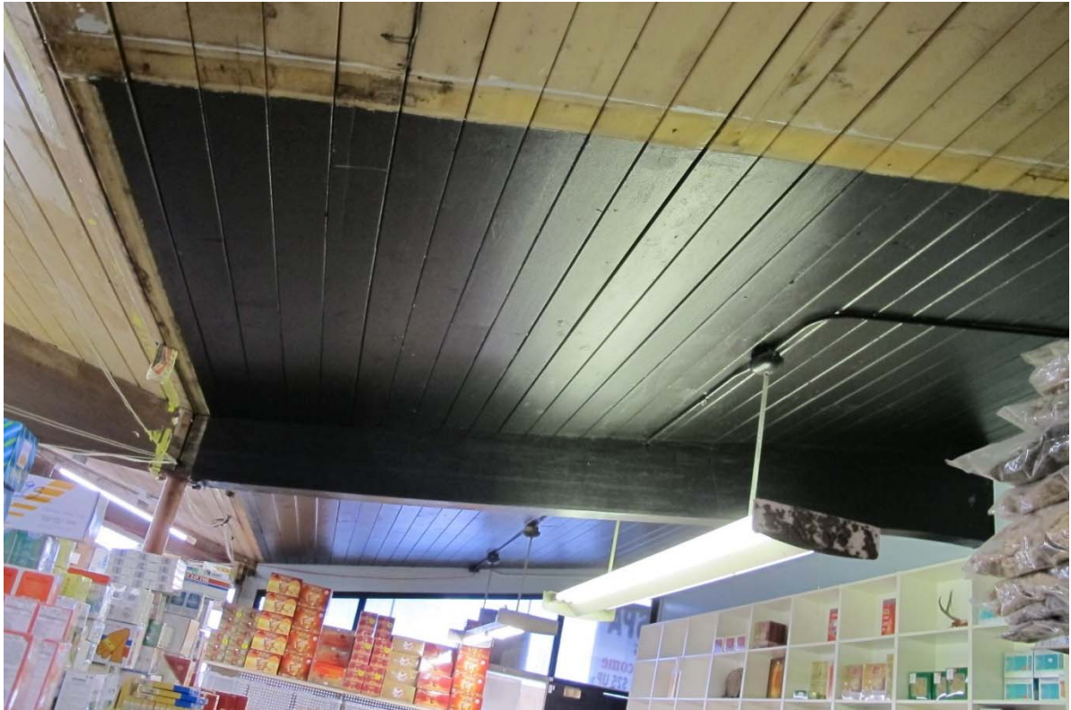
Fig. 83 – Interior, fifth bay (grocery store) at far left; fourth bay at middle and right; detail of ceiling.
