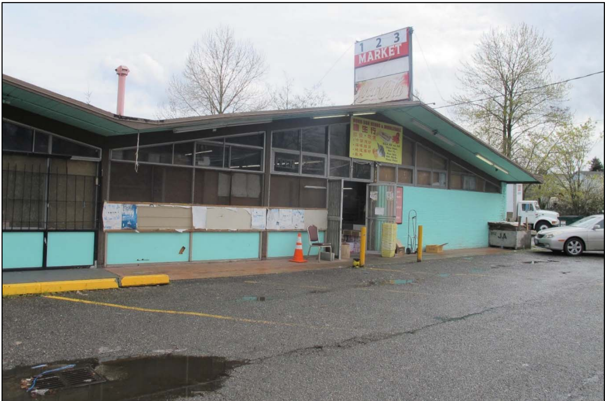
Fig. 60 – West elevation—fifth bay
