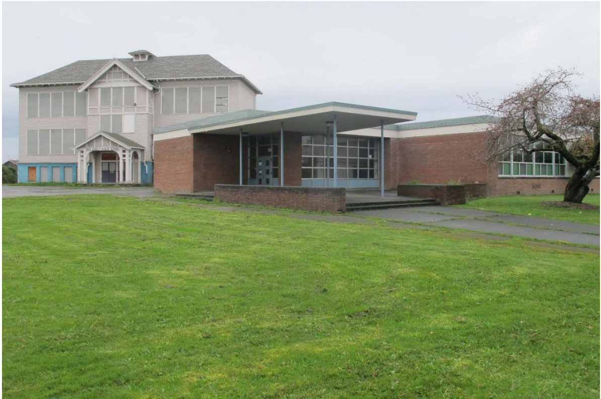
Fig. 33 – Context: Van Asselt Elementary School, across Beacon Avenue South from subject site. Old school building (Edgar Blair, 1910) at left; new building (Jones & Bindon, 1950) at right.
