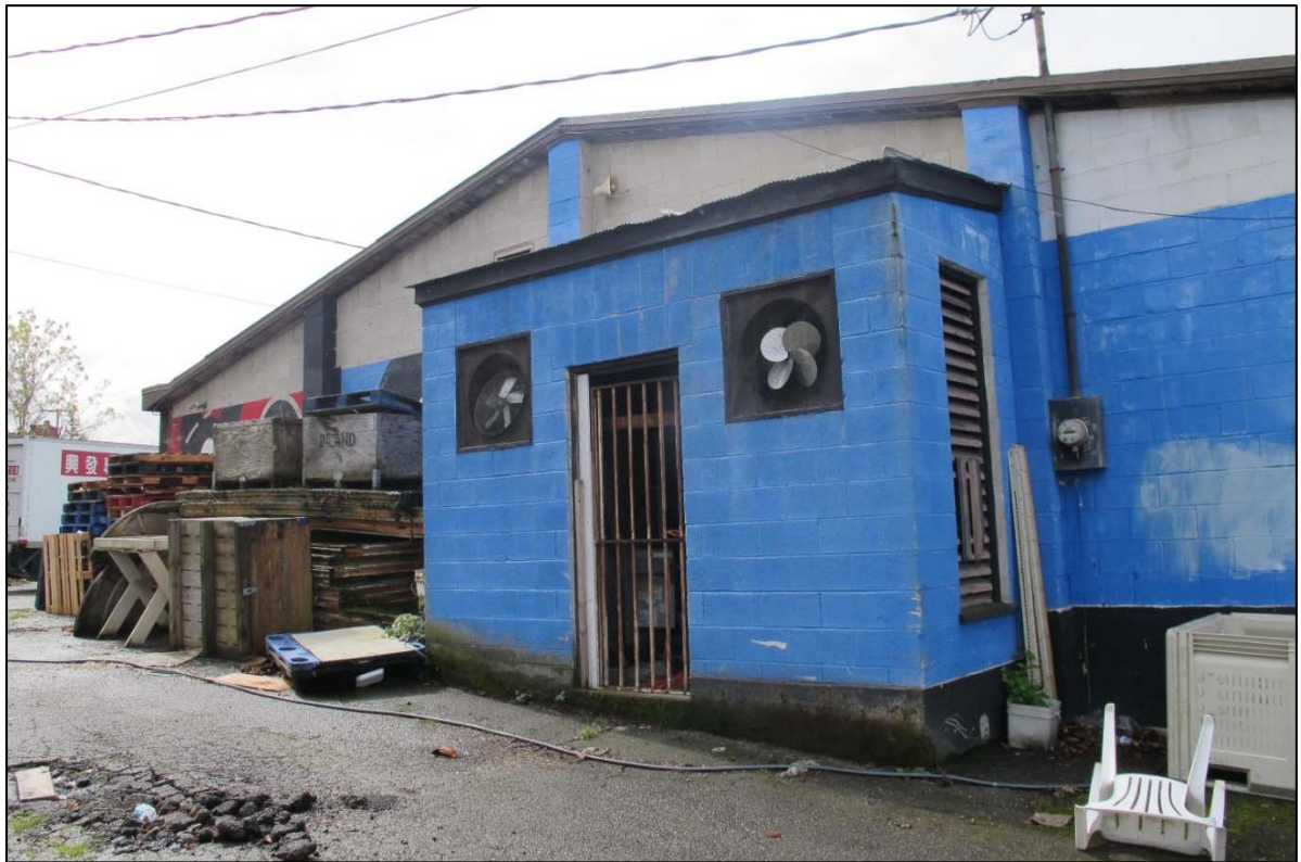
Fig. 40 – East elevation, south portion, fifth bay (largest bay containing grocery store)
