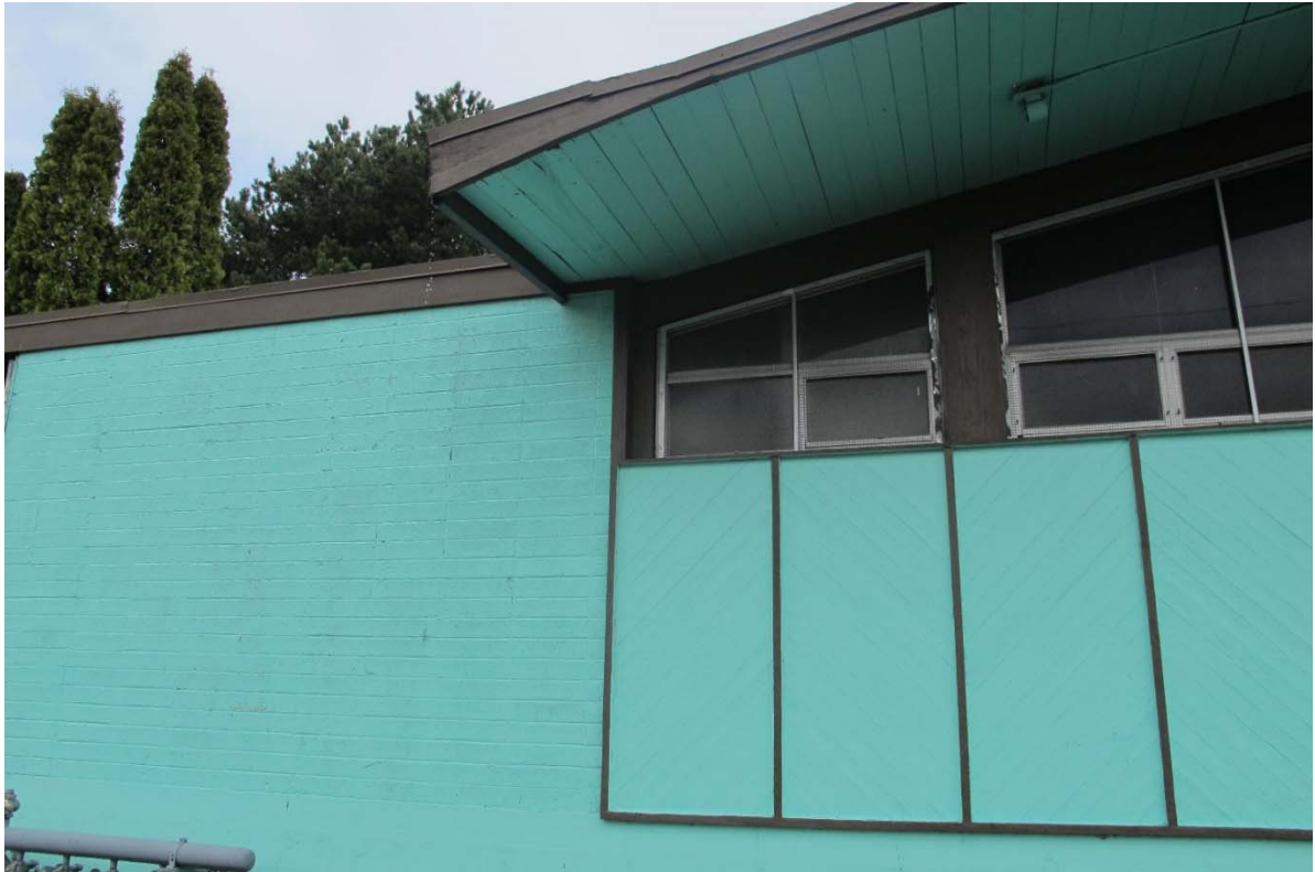
Fig. 55 – West elevation—first bay with flat roofed extension, detail
