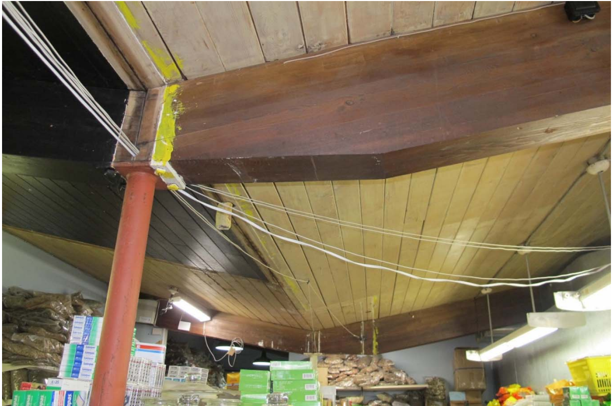
Fig. 77 – Interior, fourth and fifth bay (grocery store), detail of glue-laminated beam
