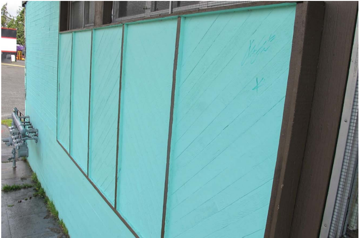
Fig. 54 – West elevation—first bay, detail of panel below window
