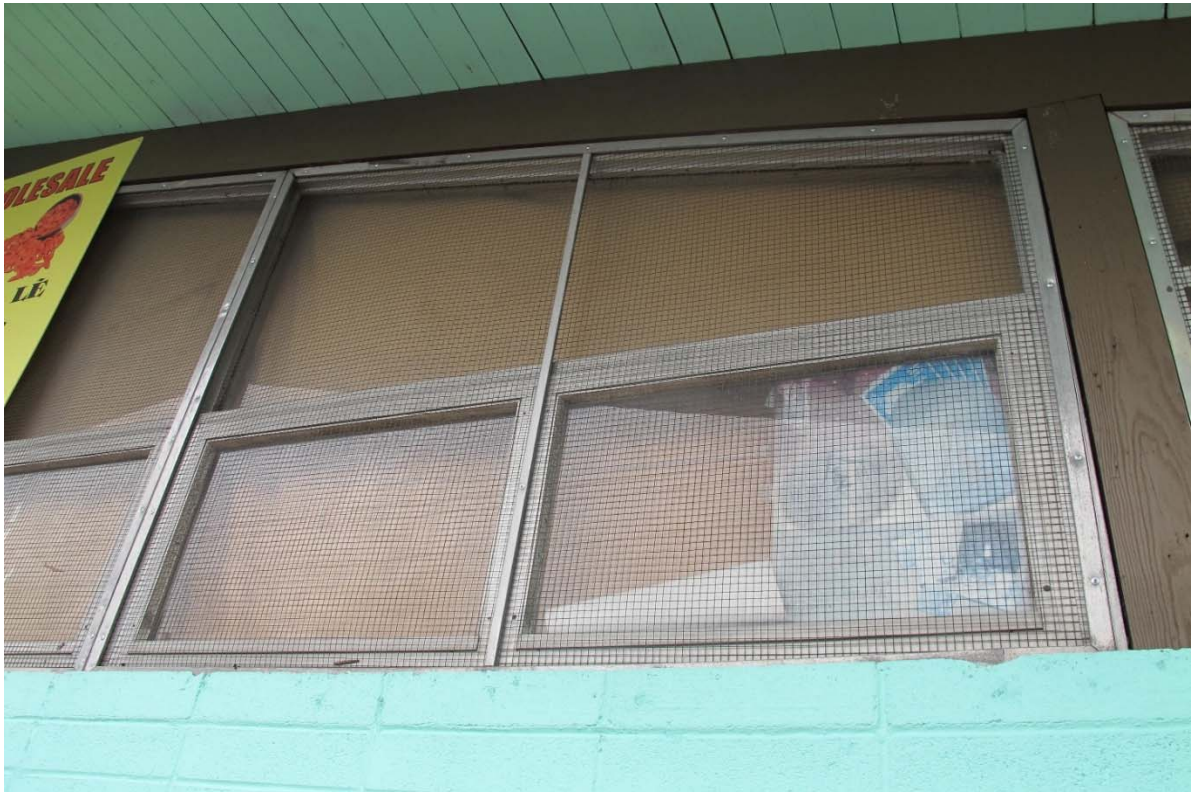
Fig. 66 – West elevation—fifth bay, detail of windows
