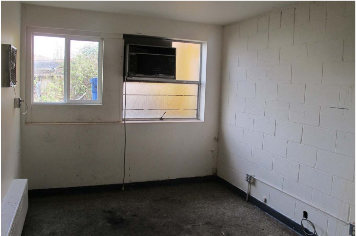
Fig. 93 – Interior, first bay (former religious facility)
