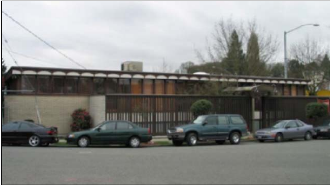
Fig. 27 – Rudy Simone Construction Company offices, 2200 Rainier Avenue S, (Richard Bouillon, 1964). (DON, 2004)
