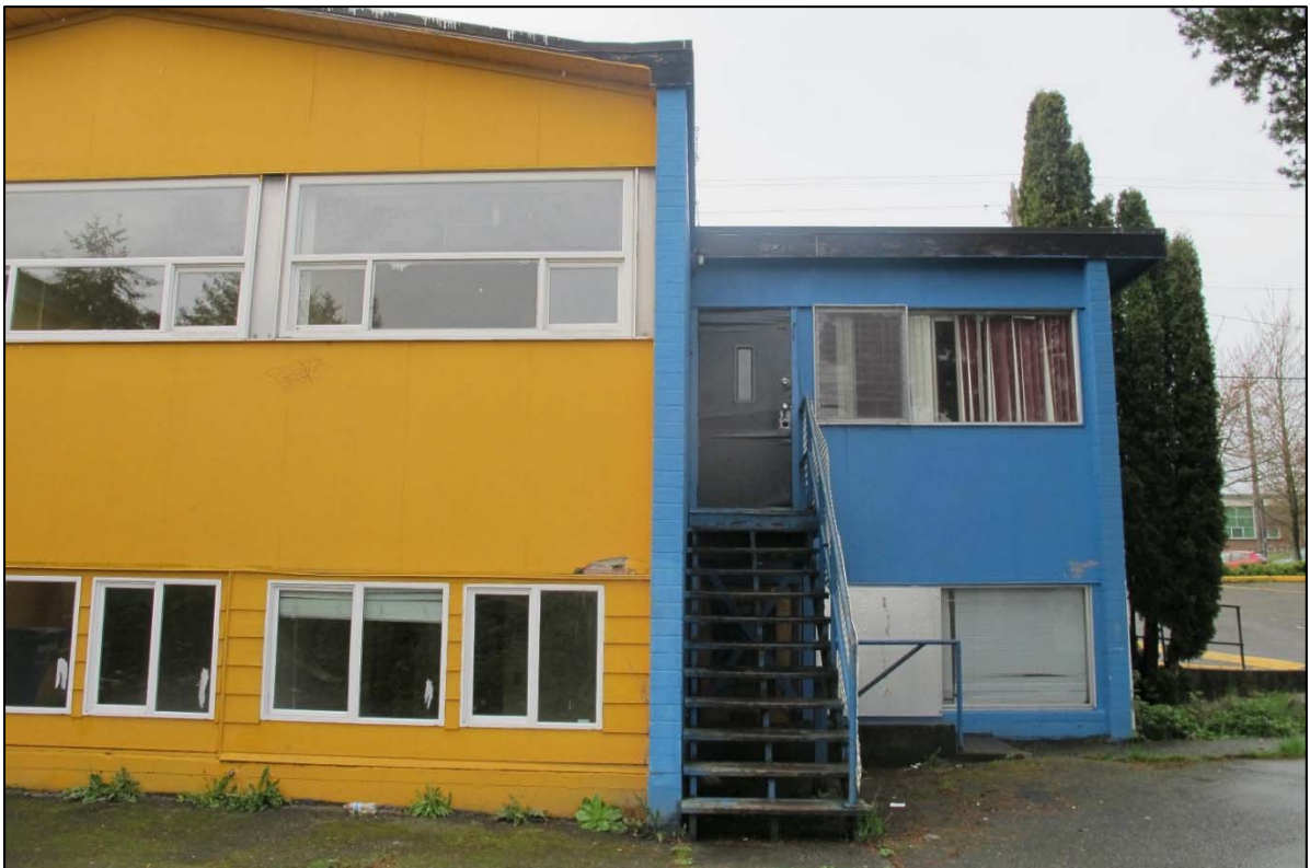
Fig. 48 – East elevation—first bay and flat roofed extension
