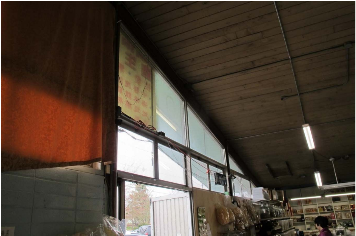
Fig. 70 – Interior, fifth bay (grocery store)
