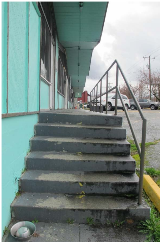
Fig. 62 – West elevation—first bay, view southward at exterior steps
