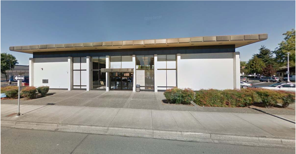
Fig. 20 – First Federal Savings & Loan, 858 S. Second Street, Renton (Benjamin Woo, 1967) (Google Streetview)
