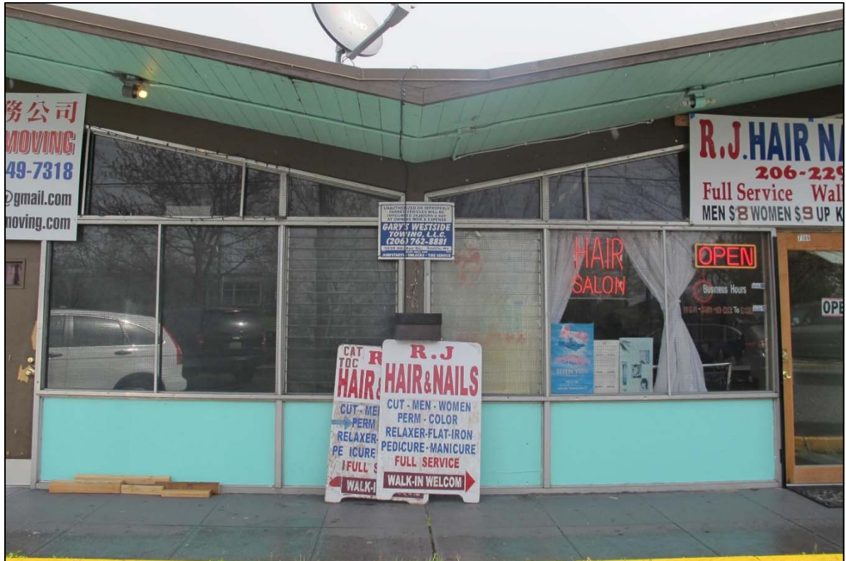
Fig. 61 – West elevation—third and fourth bay, detail
