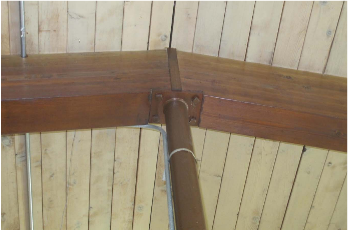
Fig. 73 – Interior, fifth bay (grocery store), detail of metal column and glue-laminated beam
