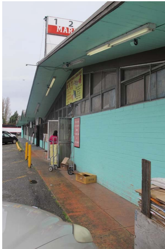
Fig. 68 – West elevation—fifth bay, detail
