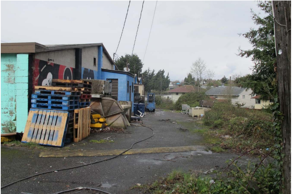
Fig. 39 – East elevation, view from south
