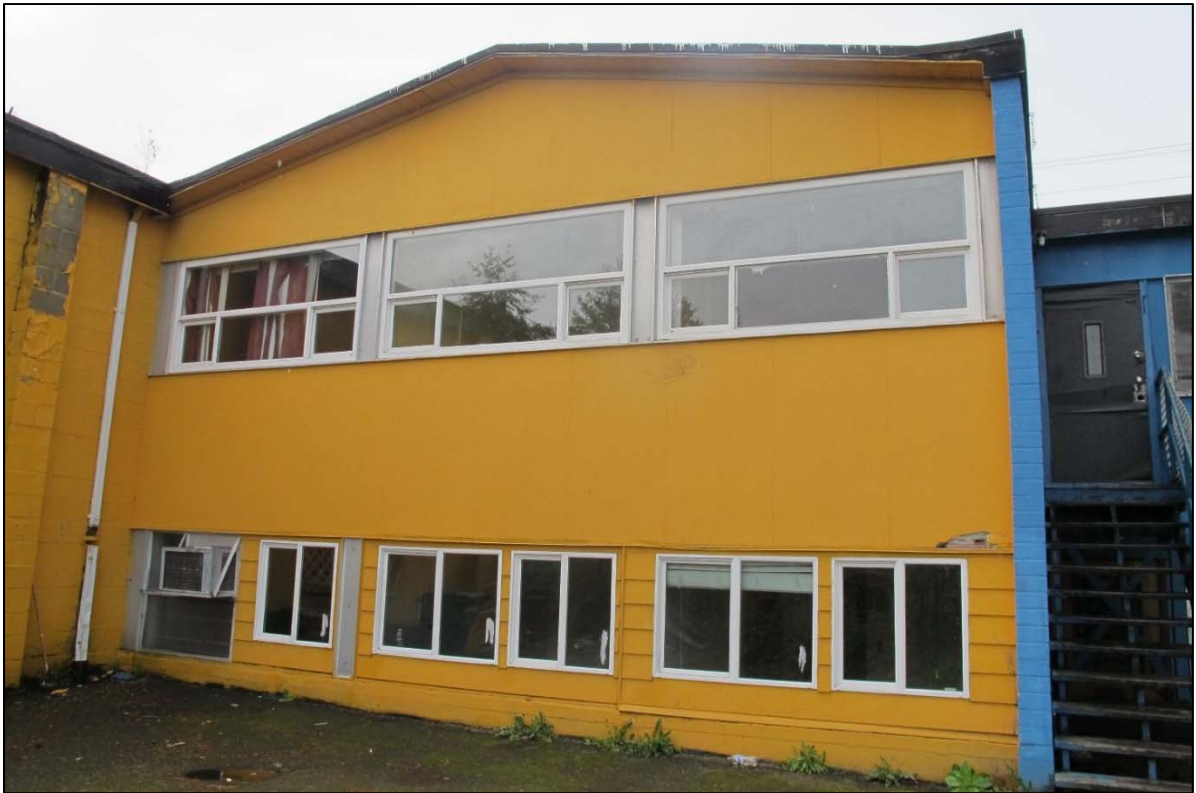
Fig. 47 – East elevation—first bay
