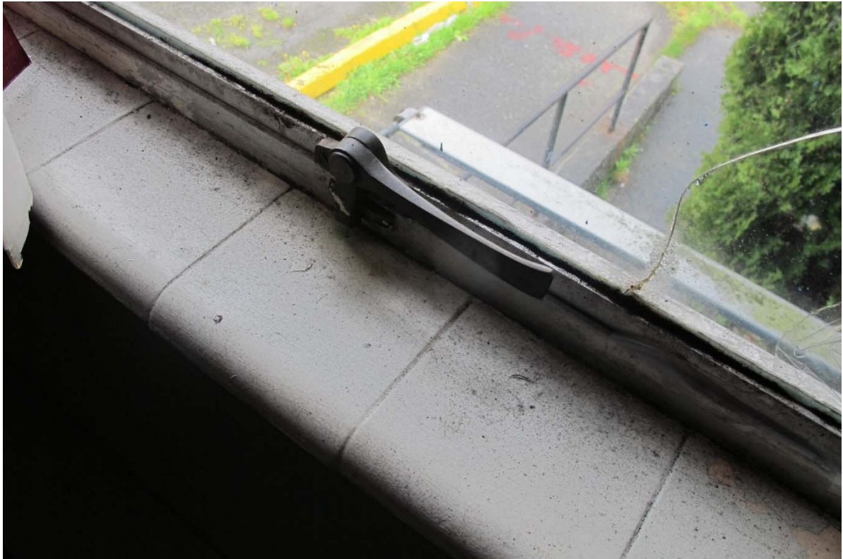
Fig. 91 – Interior, first bay (former religious facility), detail of window sill and hardware
