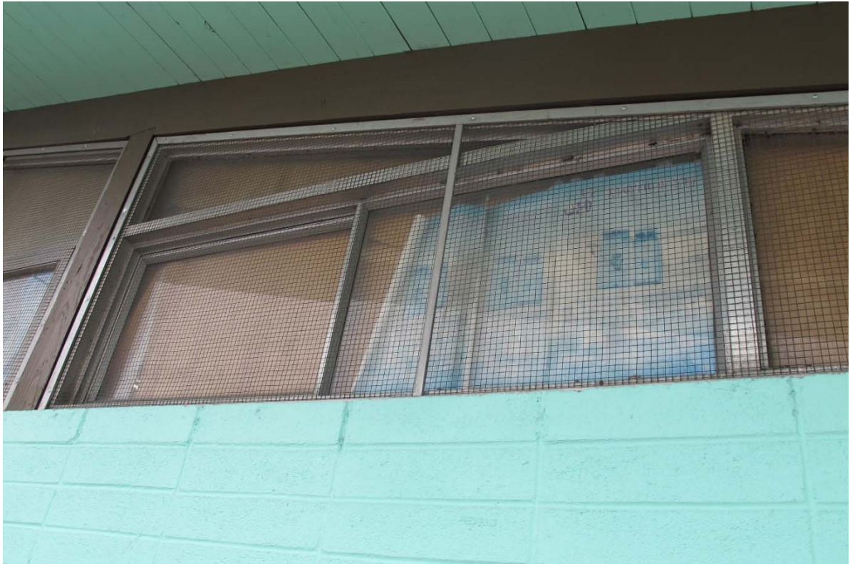
Fig. 65 – West elevation—fifth bay, detail of windows
