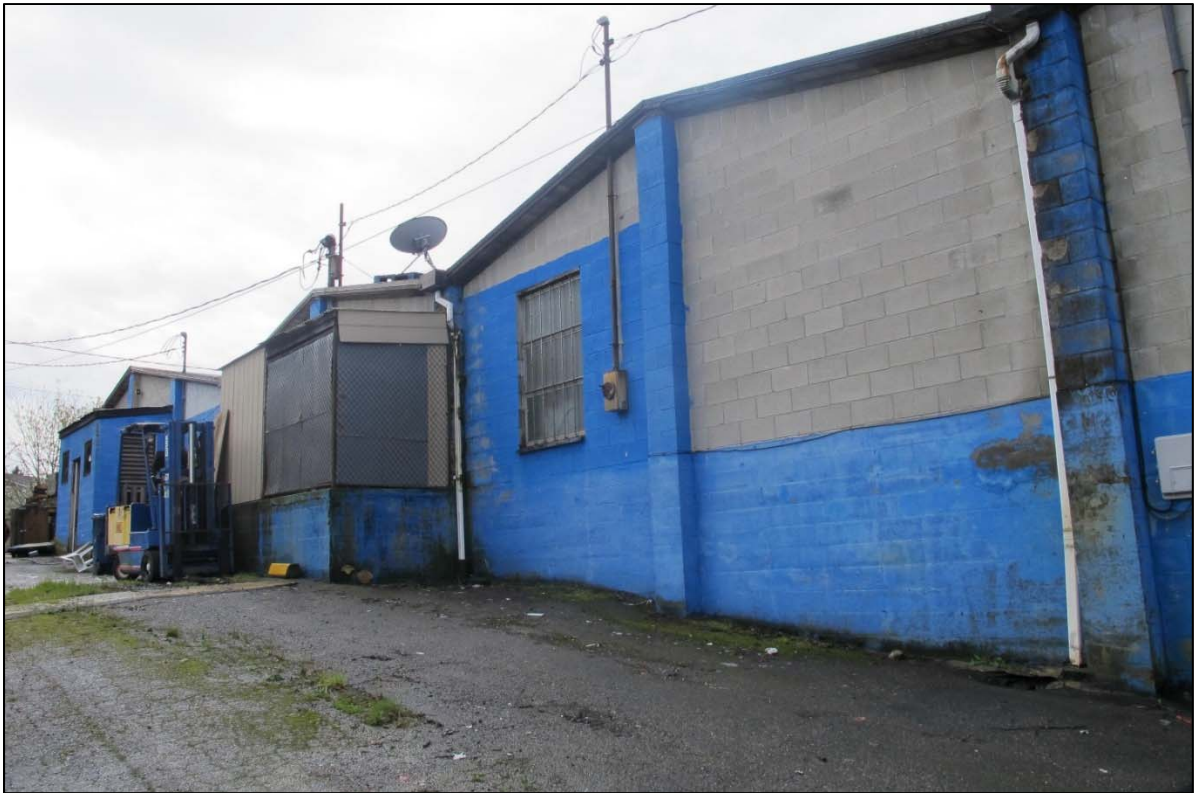
Fig. 43 – East elevation—fifth, fourth, third bays
