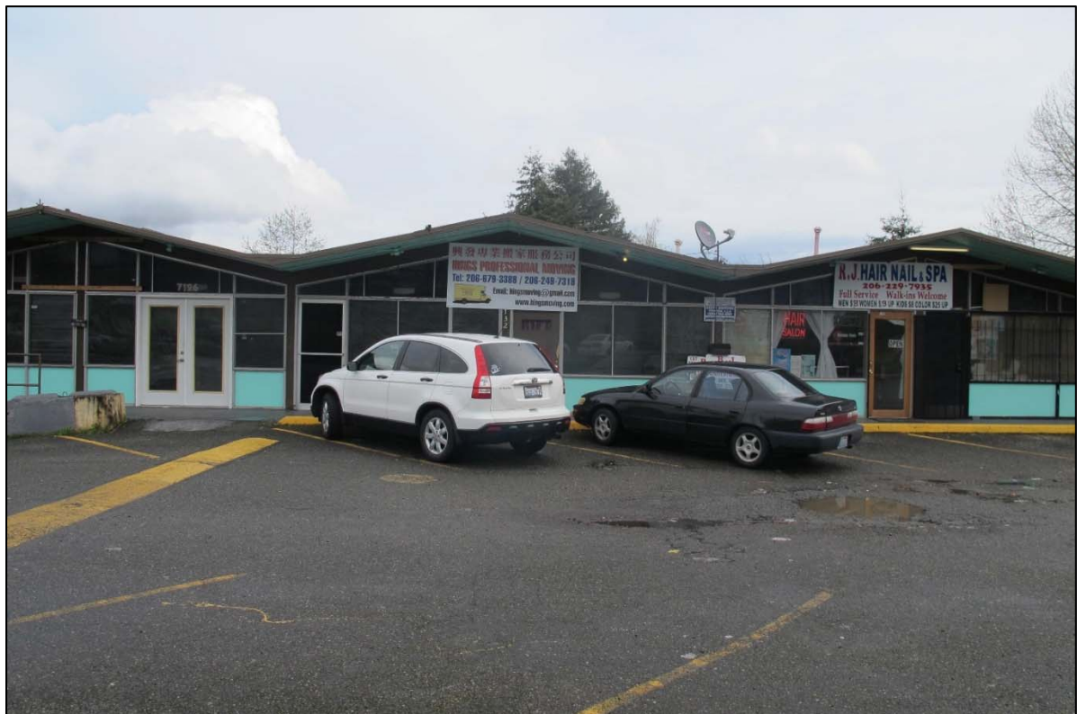
Fig. 58 – West elevation—second, third, and fourth bays
