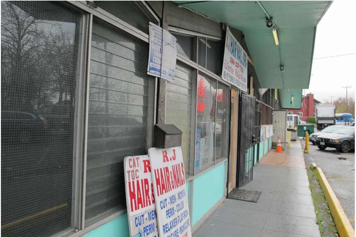
Fig. 67 – West elevation—view southward along front walk
